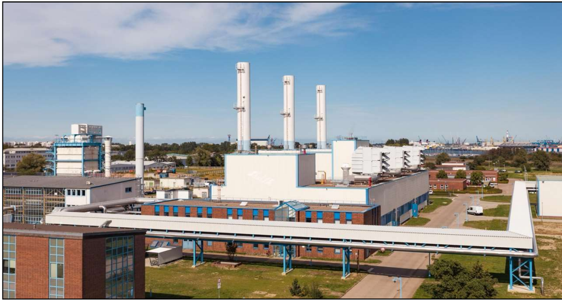
Figure 3.27: Combined cycle gas turbine (CCGT) plant in Marienehe.
