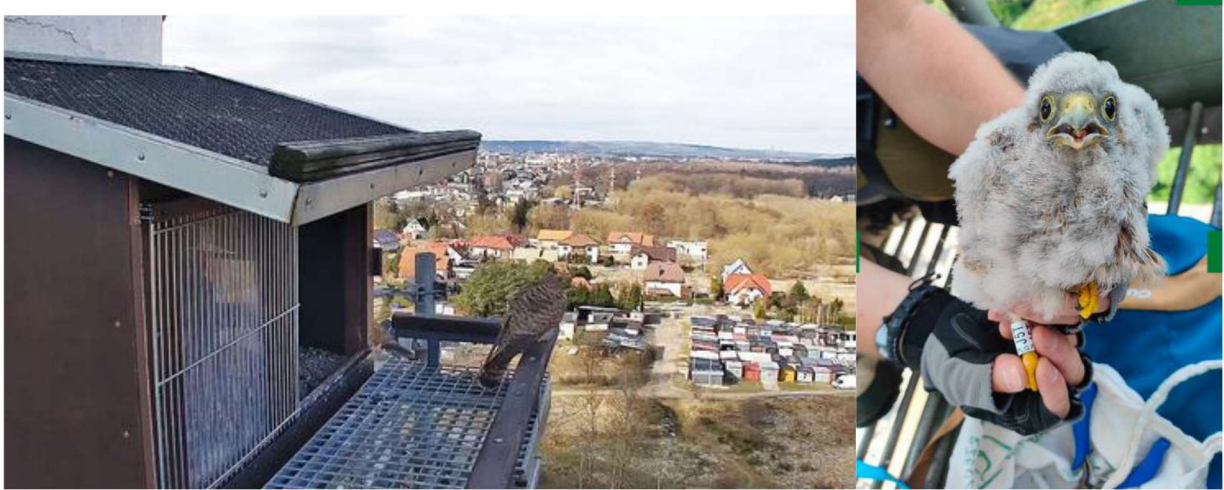
Figure 3.16: An artificial nest for kestrel falcons in the Wejherowo heating plant.
